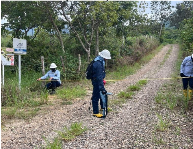
FIGURE 1: RIGHT OF WAY ROUTE PATROL
