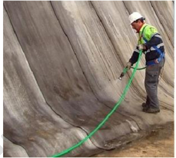
FIGURE 5. Concrete mats for slope protection. Source: Internet (2020).
