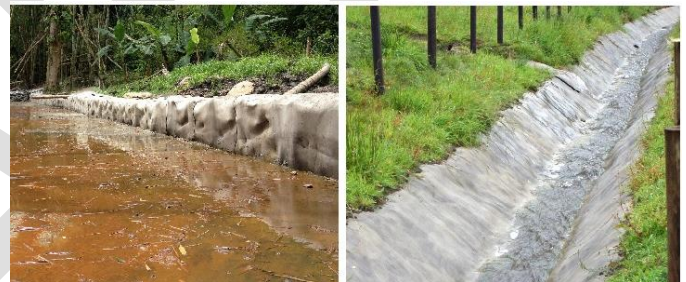
FIGURE 6. Concrete mats for water control. Source: Internet (2020).
