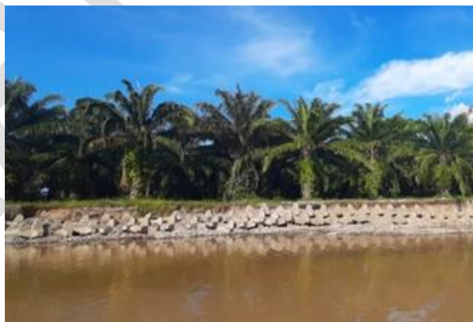
FIGURE 2. Riverbank defense with concrete blocks. Source: Internet (2020).
