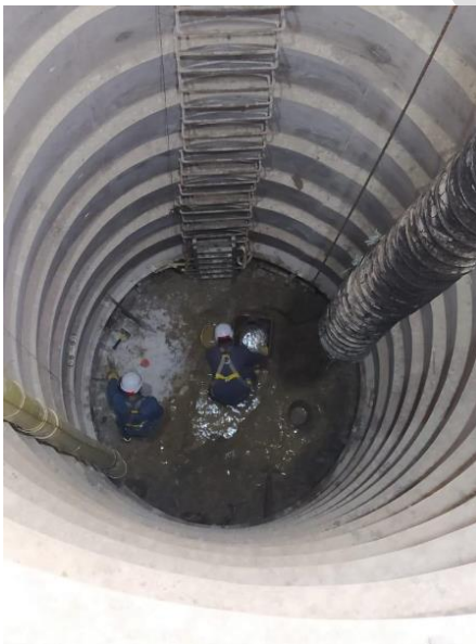
FIGURE 4. Horizontal drain collection chamber for piezometric level reduction. Source: Internet (2020).
