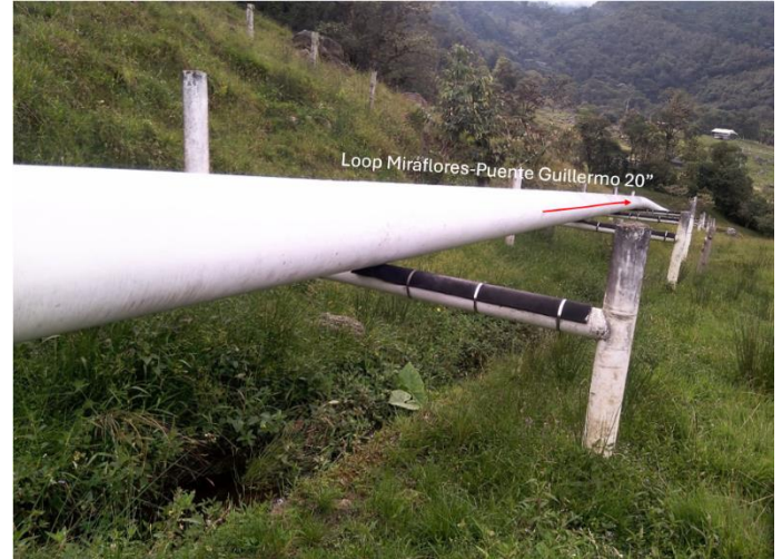
FIGURE 1: Location of the 20" loop on H-frames
