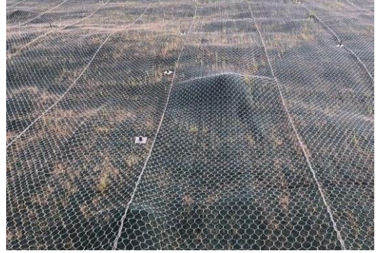
FIGURE 12: Example of a rock mass stabilized with mesh and bolts/anchors
