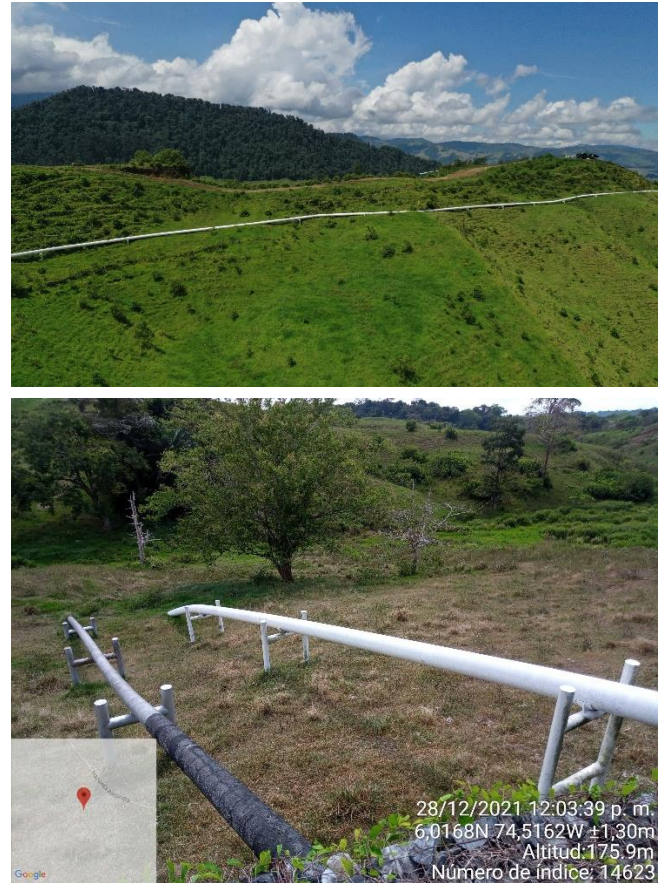
FIGURE 7: Top – Surface-level segment excluded from the analysis due to its location at the top of a slope composed of volcanic deposits, near the ridge, where the possibility of rockfall impact is null and there are no adjacent slopes contributing rocky material. Bottom – Surface-level segment excluded from the analysis for the same reason: located at the upper part of a slope with volcanic deposits, near the ridge, with no potential for rockfall impact or contributing rock sources from adjacent slopes.
