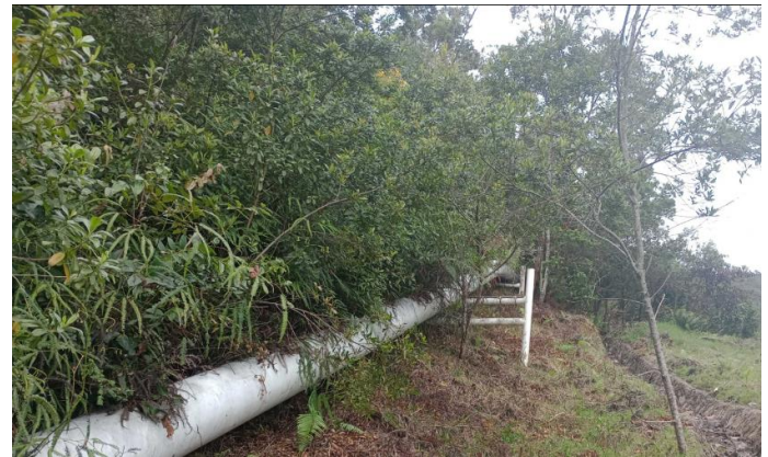
FIGURE 9: PK96+263 of the 20" Loop in the Miraflores – Puente Guillermo section, showing a 280 m slope on the left side with a 21^\circ gradient and dense vegetation cover, where block displacement is not possible.
