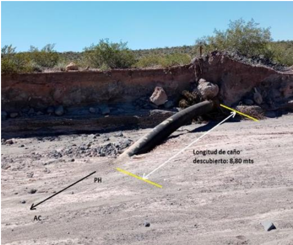
FIGURE 2 – Exposed pipeline – Source: Author of the paper
