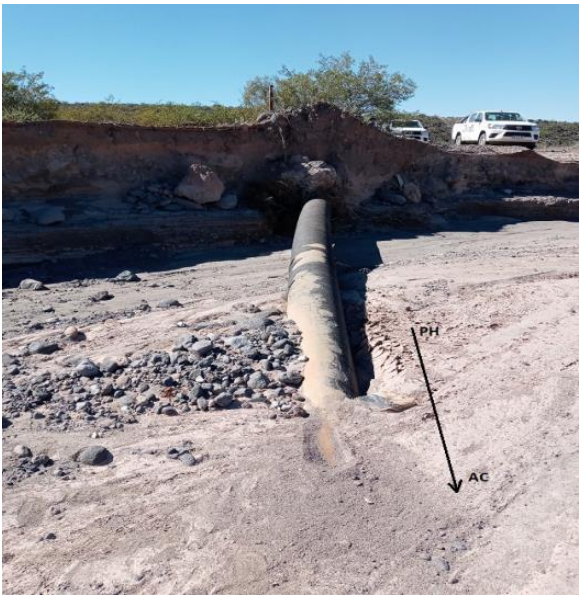
FIGURE 3 – Exposed pipeline – Source: Author of the paper
