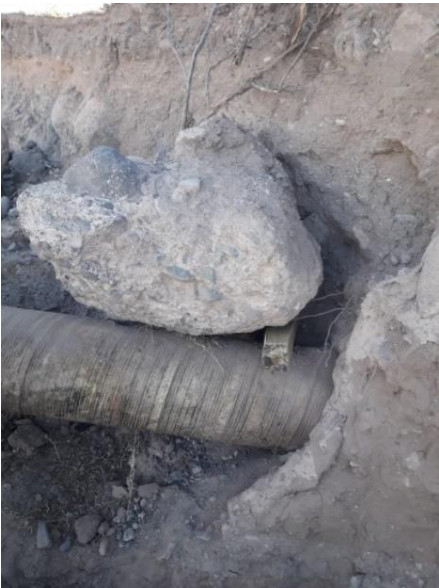
FIGURE 9 - Stone on the pipeline after the event - Source: Author of the paper
