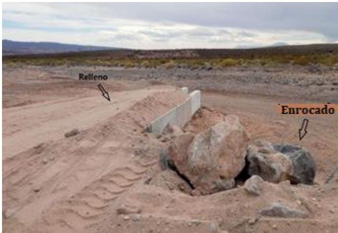
FIGURE 27 – Materialization of erosion protection rocks - Source: Author of the paper
