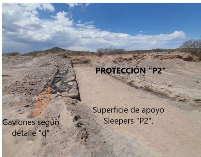
FIGURE 21 – Preparation of inclined surface for the placement of sleepers - Source: Author of the paper
