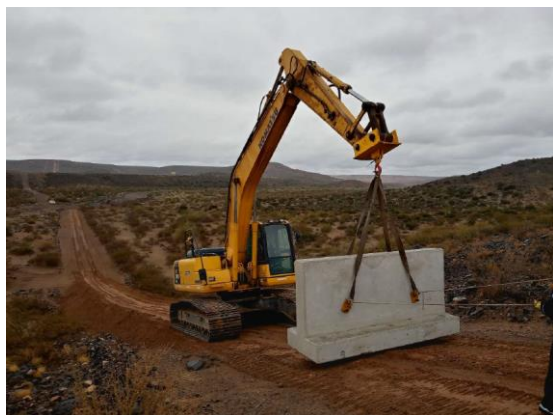
FIGURE 19 – Equipment moving a sleeper – Source: Author of the paper
