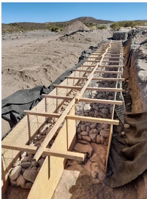
FIGURE 20 – Construction of foot protections to prevent undermining - Source: Author of the paper
