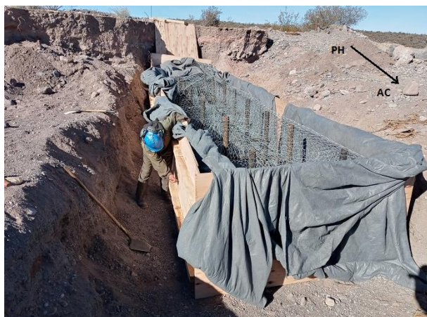
FIGURE 16 – Construction of temporary work with gabions and reinforcement tubing – Source: Author of the paper
