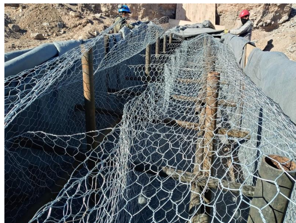
FIGURE 15 – Construction of temporary work with gabions and reinforcement tubing – Source: Author of the paper
