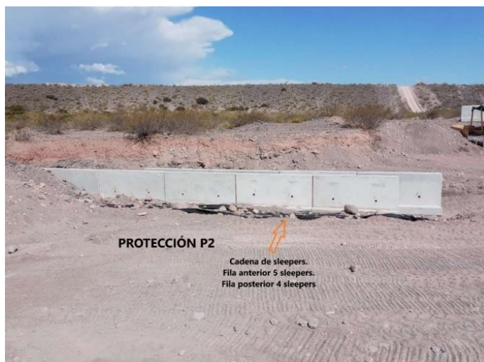
FIGURE 22 – Sleepers in final position - Source: YPF SA
