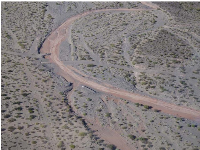
FIGURE 32 Aerial view of completed work 3 – Source: YPF SA
