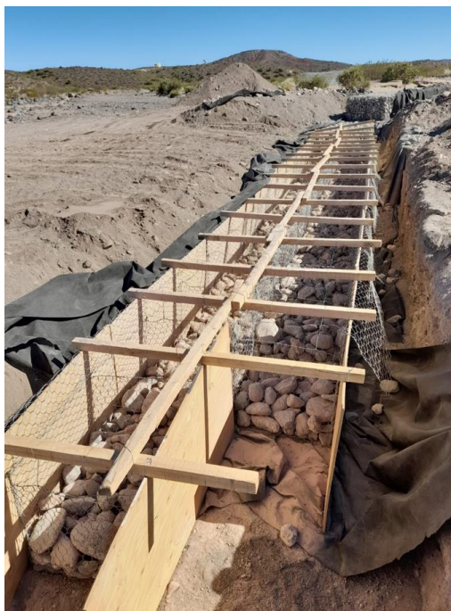
FIGURE 20 – Construction of foot protections to prevent undermining - Source: YPF SA
