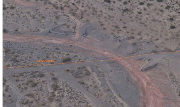
FIGURE 33 - Aerial view of completed work with relative location of the pipeline - Source: YPF SA
