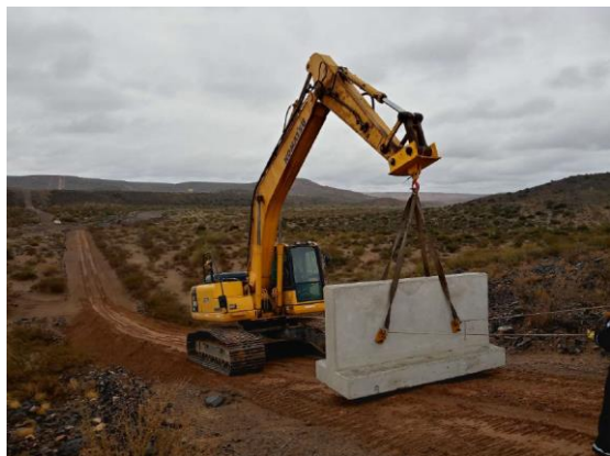
FIGURE 19 – Equipment moving a sleeper – Source: YPF SA
