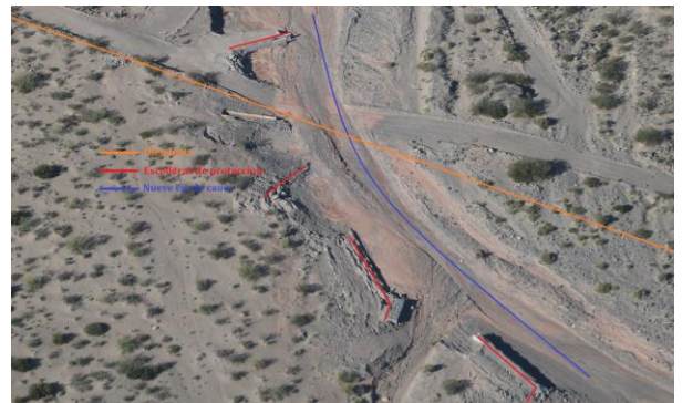
FIGURE 30 – Aerial view of completed work 1 – Source: YPF SA
