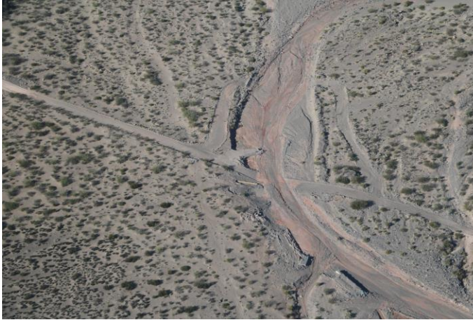
FIGURE 31 – Aerial view of completed work 2 - Source: YPF SA
