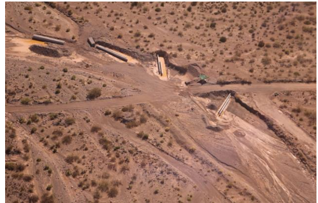
FIGURE 25 – Aerial view of the construction site - Source: YPF SA
