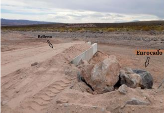
FIGURE 27 – Materialization of erosion protection rocks - Source: YPF SA
