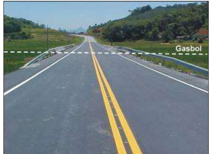
FIGURE 25: PROTECTION WITH VIADUCT OVER BORED PILES CONCLUDED.
