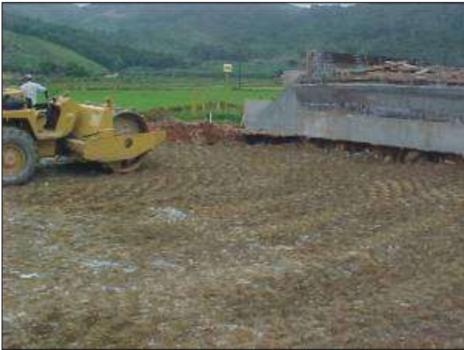
FIGURE 23: SOFT SOIL EXCAVATION CLOSE TO BORED PILE WALL.
