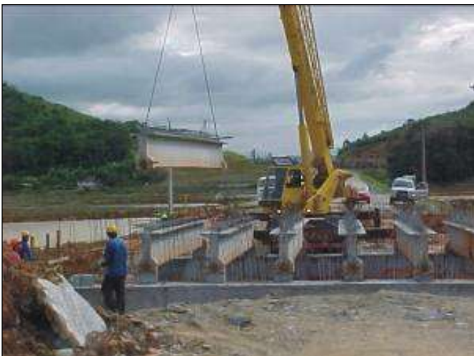
FIGURE 24: VIADUCT BEAMS INTALLATION.
