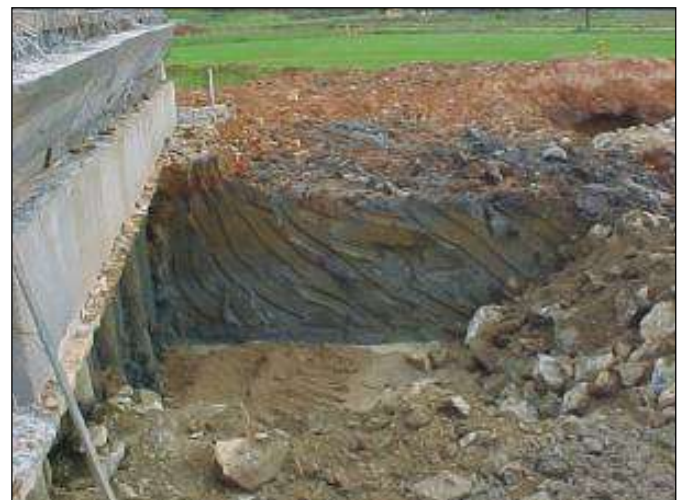
FIGURE 22: SOFT SOIL EXCAVATION CLOSE TO BORED PILE WALL.
