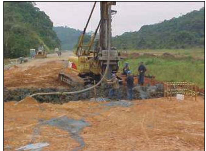
FIGURE 21: BORED PILES EXECUTION.
