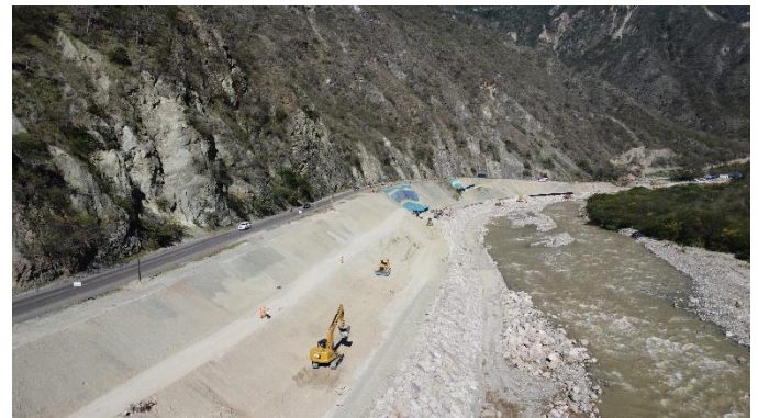
FIGURE 25: CONSTRUCTION PROCEDURE FOR TERRACE FILING.
