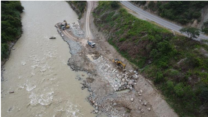
FIGURE 11: CONSTRUCTIVE PROCEDURE OF RIPRAP.
