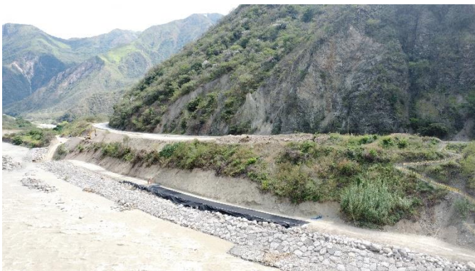
FIGURE 18: CONSTRUCTION PROCEDURE FOR GEOTEXTILE INSTALLATION.
