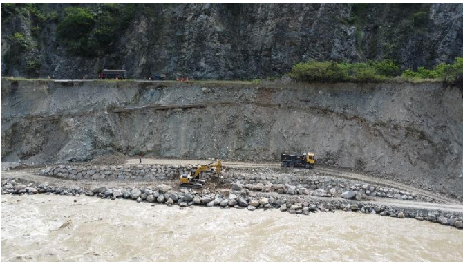
FIGURE 22: CONSTRUCTIVE PROCEDURE OF REAR FILL OF RIPRAP.
