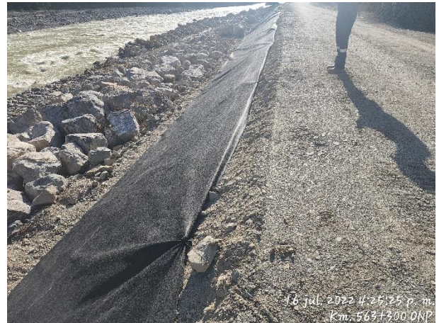
FIGURE 19: CONSTRUCTION PROCEDURE FOR GEOTEXTILE INSTALLATION.
