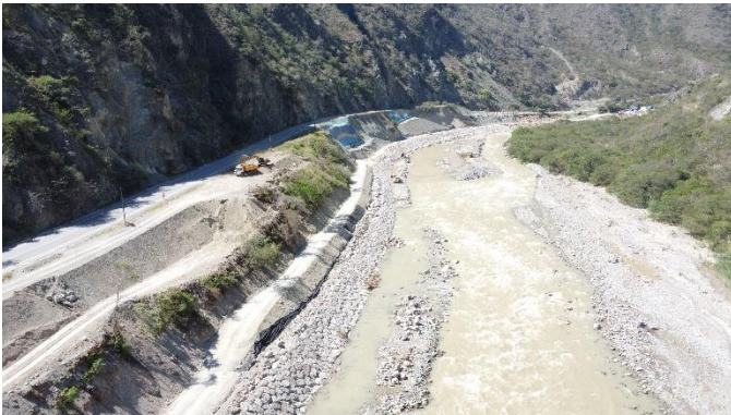
FIGURE 21: CONSTRUCTIVE PROCEDURE OF REAR FILL OF RIPRAP.
