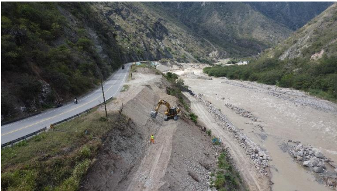
FIGURE 27: CONSTRUCTIVE PROCEDURE OF CUTE FOR TERRACE.
