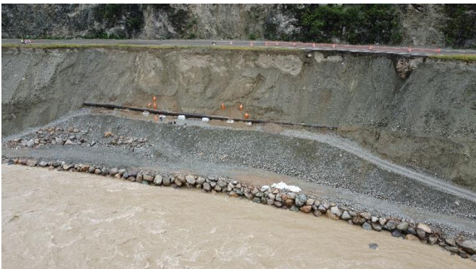
FIGURE 23: FILTER LAYER PLACEMENT CONSTRUCTIVE PROCEDURE.
