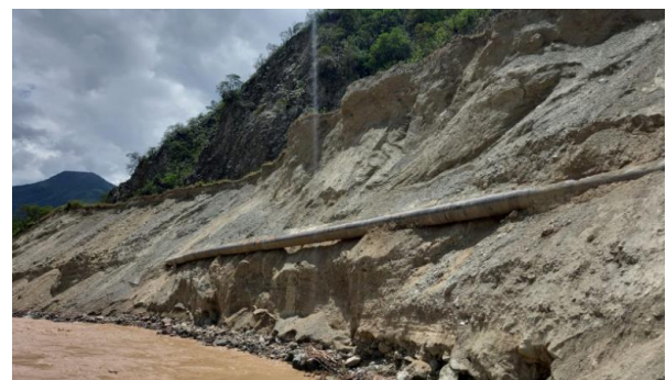
FIGURE 2: SECTOR 1 OF 58 METERS OF 36" PIPE WAS FULLY EXPOSED.
