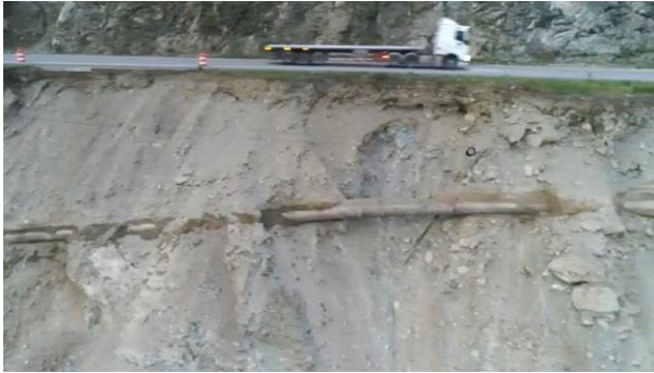
FIGURE 3: SECTOR 2 OF 41 METERS OF 36” PIPE WAS FULLY EXPOSED.
