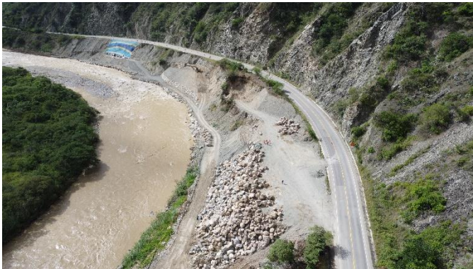
FIGURE 16: ROCKFILL CONSTRUCTIVE PROCEDURE FOR RIPRAP.
