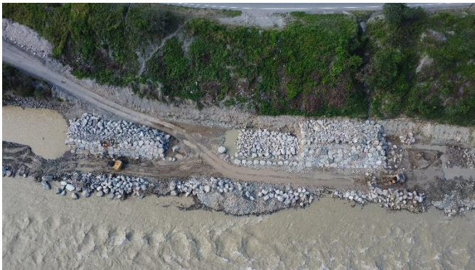
FIGURE 17: ROCKFILL CONSTRUCTIVE PROCEDURE FOR RIPRAP.
