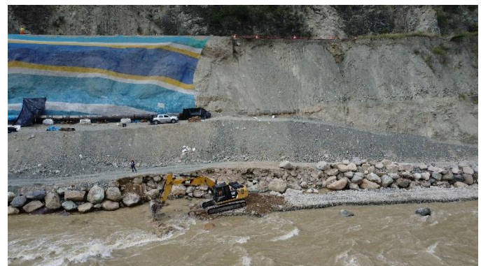
FIGURE 9: CONSTRUCTIVE PROCEDURE OF RIPRAP.
