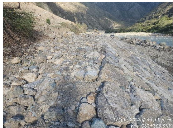
FIGURE 15: CONSTRUCTIVE PROCEDURE OF RIPRAP.
