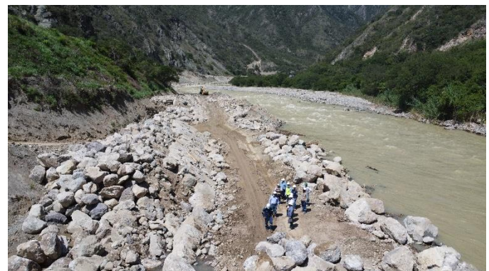
FIGURE 10: CONSTRUCTIVE PROCEDURE OF RIPRAP.
