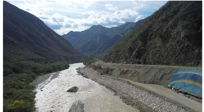
FIGURE 14: CONSTRUCTIVE PROCEDURE OF RIPRAP.
