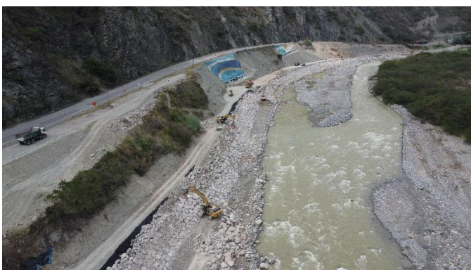
FIGURE 13: CONSTRUCTIVE PROCEDURE OF RIPRAP.
