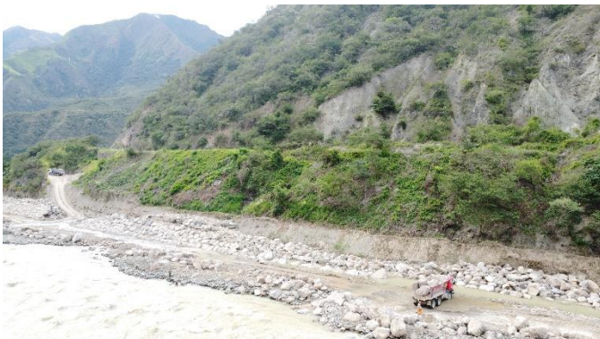
FIGURE 12: CONSTRUCTIVE PROCEDURE OF RIPRAP.
