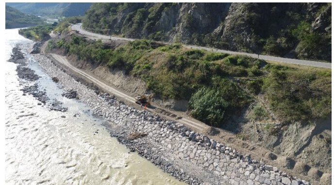
FIGURE 20: CONSTRUCTIVE PROCEDURE OF REAR FILL OF RIPRAP.
