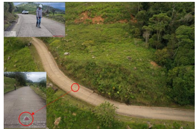
FIGURE 10. SURFACE DETECTION AND MARKING OF PIPELINE ALIGNMENT.
