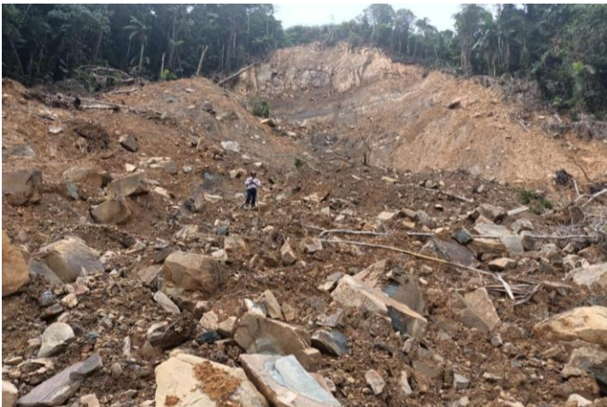
FIGURE 6. ROCK FALL AT THE TOE OF MAIN SCARP.
