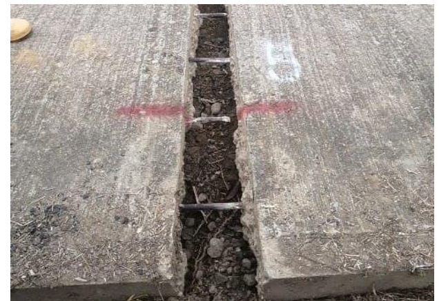
FIGURE 11. MONITORING OF THE OPENING IN CONCRETE PAVEMENT SLABS JOINTS.
