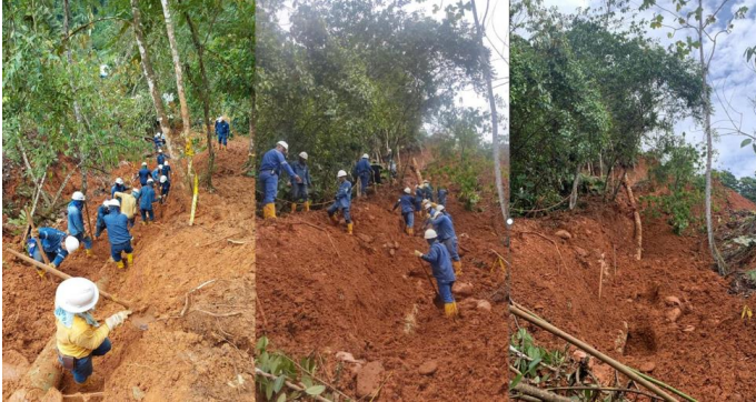
FIGURE 8. MANUAL EXCAVATION TO STRESSES RELIEF
