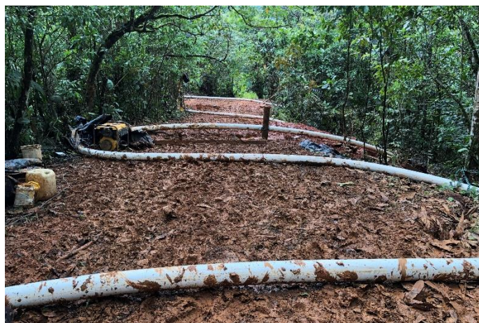
FIGURE 17. FLEXIBLE PIPE ON NARROW RIDGE
