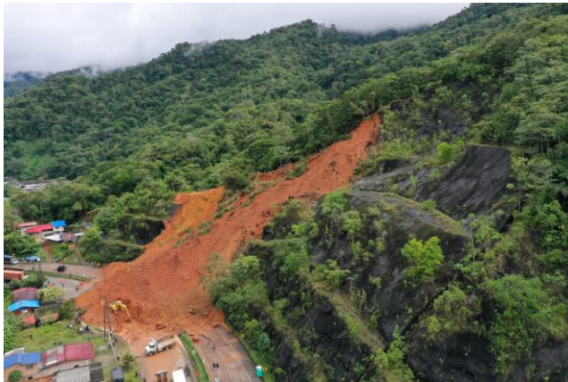
FIGURE 9. LANDSLIDE OVERVIEW AFTER CROWN COLLAPSE
