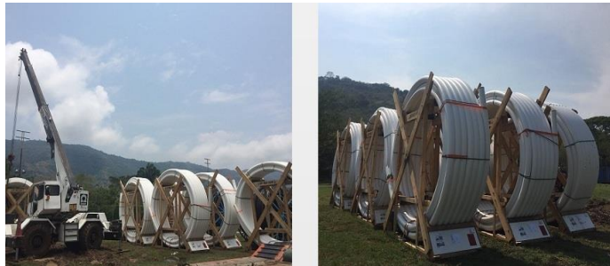
FIGURE 14. FLEXIBLE PIPE SPOOLS
