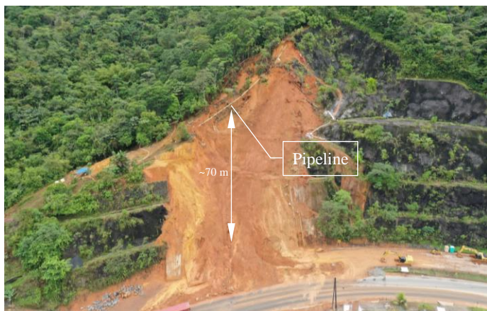
FIGURE 13. PIPELINE CONDITION AFTER LANDSLIDE RETROGRESSION
