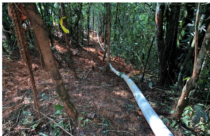
FIGURE 16. FLEXIBLE PIPE HALFWAY UP THE SLOPE
