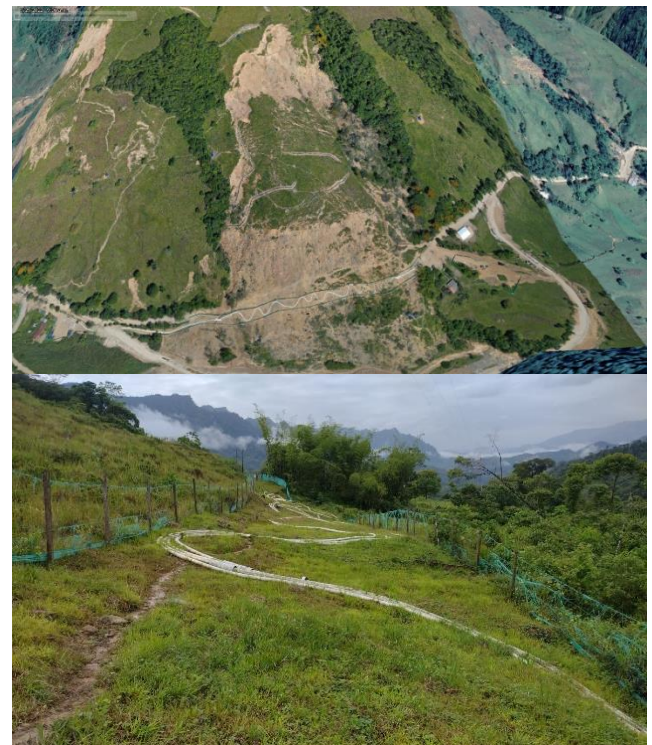
FIGURE 13: FLEXIBLE PIPE FINAL DISPOSITION.
