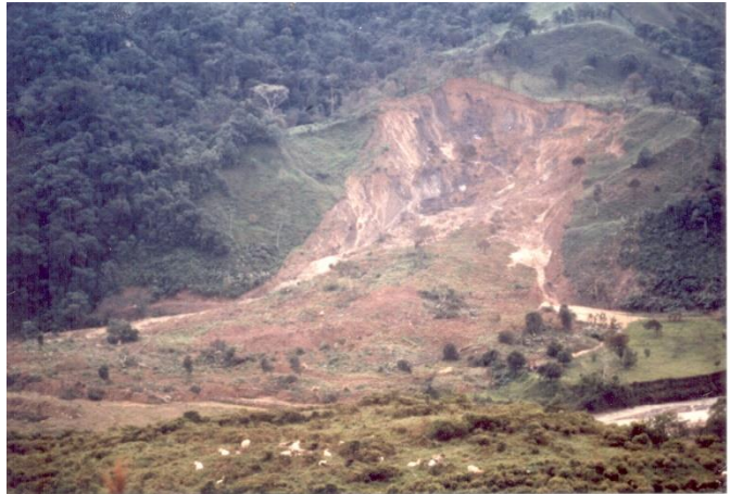
FIGURA 3: LANDSLIDE OF 1993, NOTE HOW MATERIAL FLOWED OVER ALLUVIAL DEPOSIT CAUSING PIPELINE TO COME ABOVE GROUND DUE TO LATERAL DISPLACEMENT (Photography by José Vicente Amórtegui IGL).
