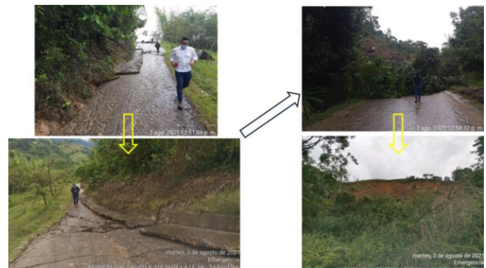
FIGURE 9: LANDSLIDE SEQUENCE THAT COVERS “LA SOBERANÍA” ROAD (Photographs by road Operator).
